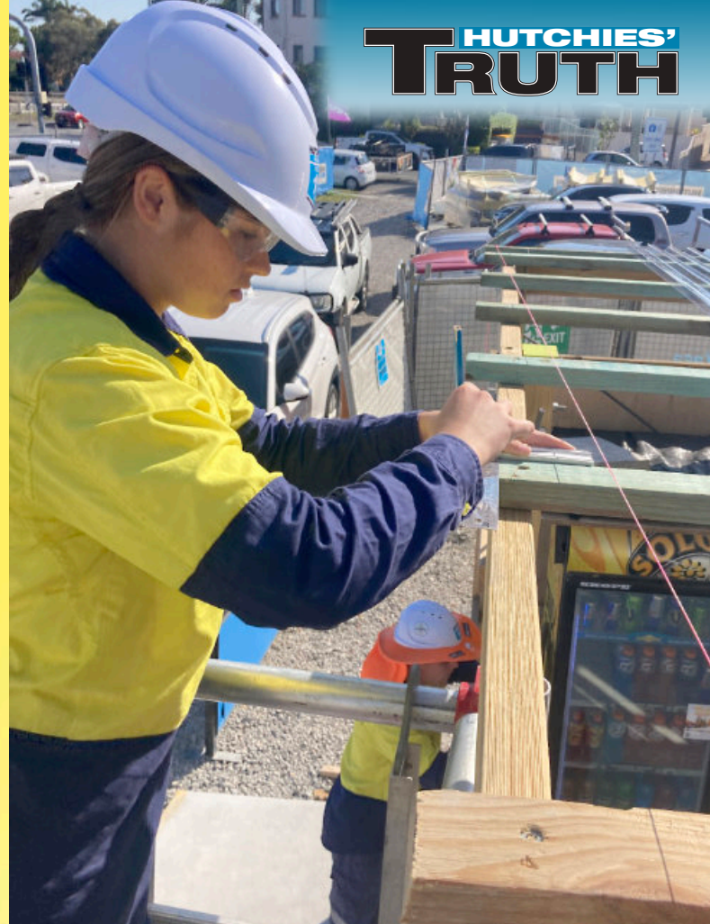
Libby at work on site.
