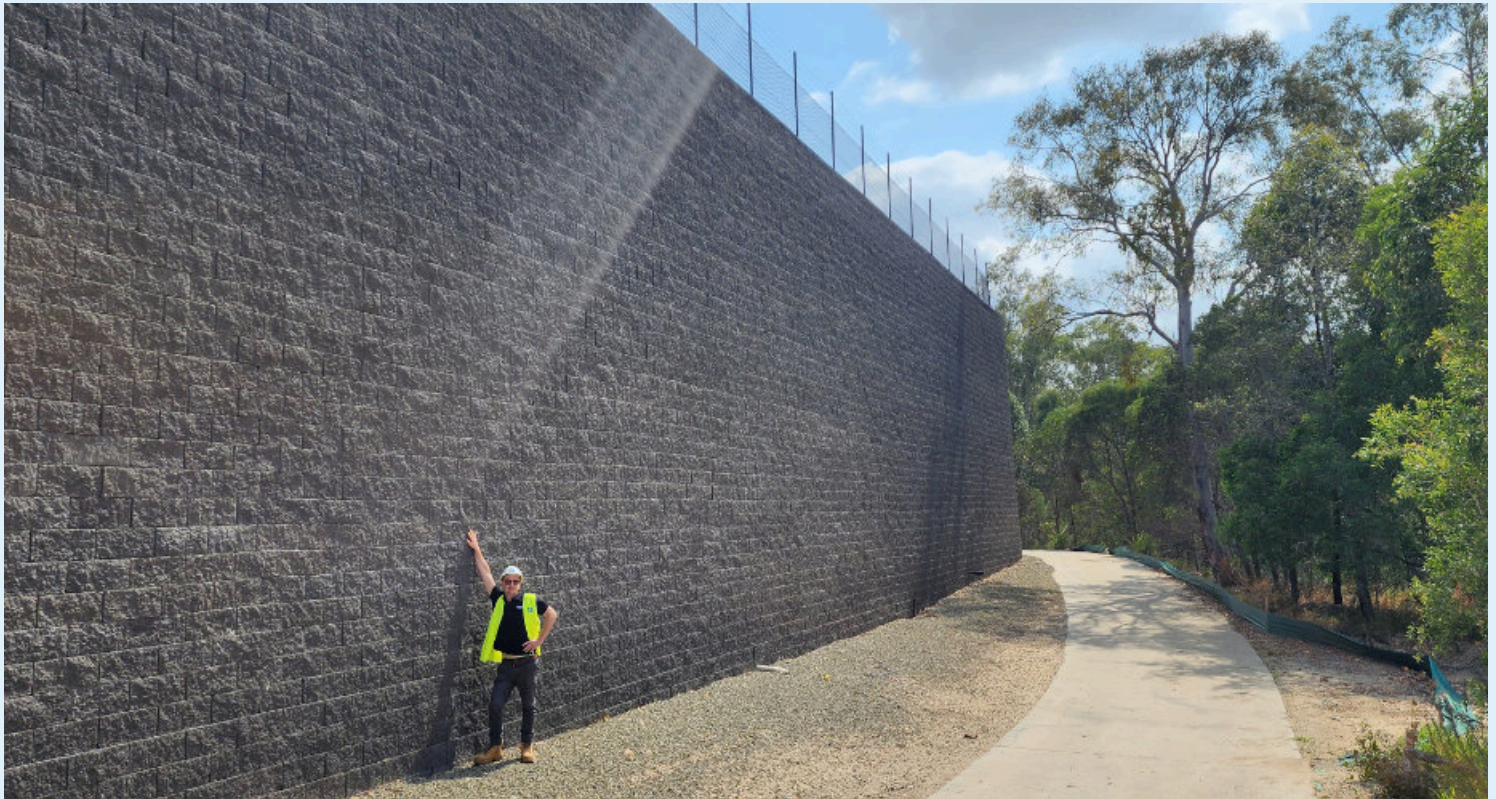
Hutchies' Luke Giles is dwarfed standing next to the impressive towering retaining wall on the Barracks Road, Wacol site – part of stage two of the Barracks at Metroplex industrial estate. The wall stretches for 1,300 metres and stands 12 metres high in some sections.
