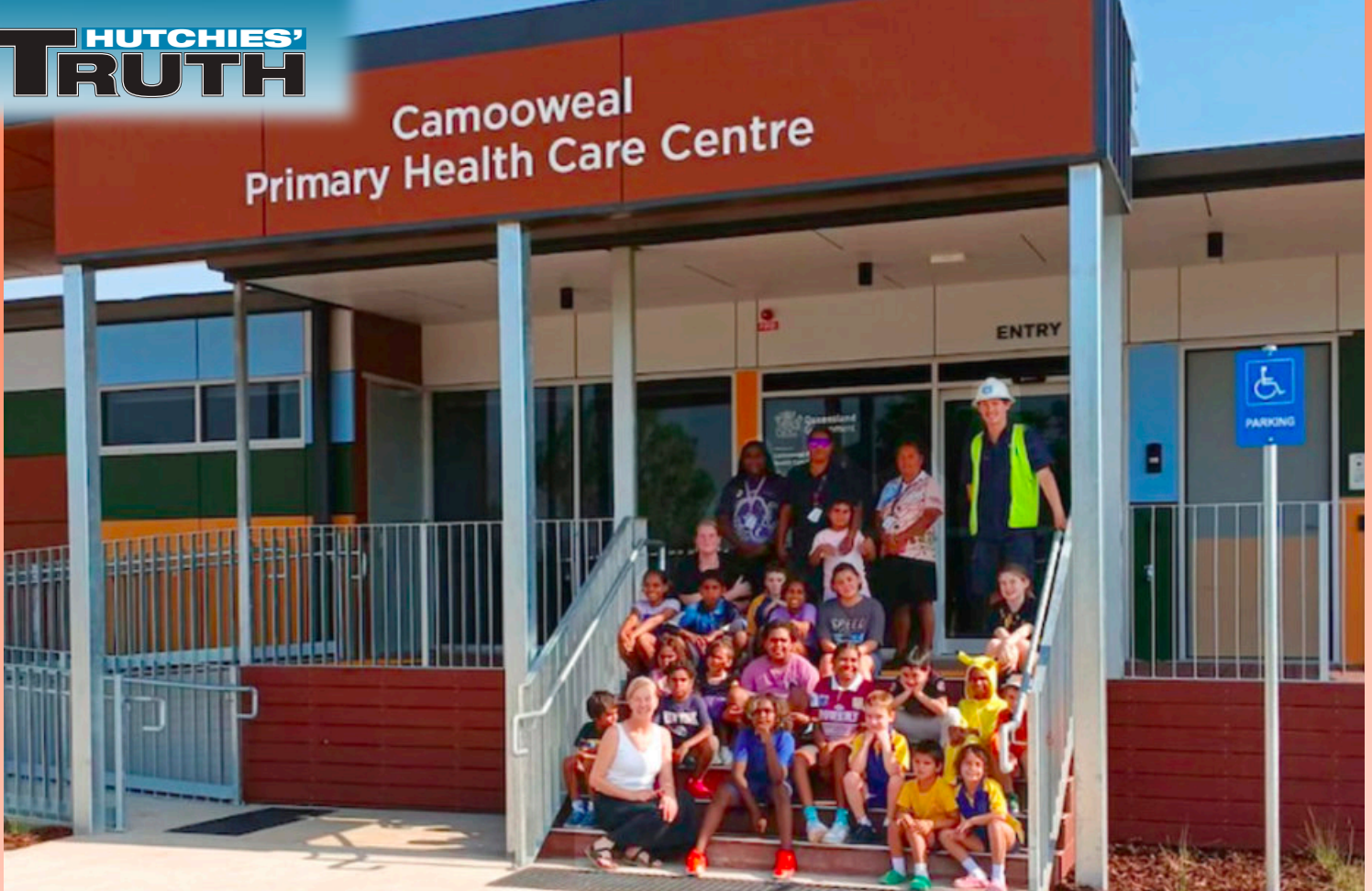
Camooweal State School students were excited to inspect their town's new hospital – under construction by Hutchies who built the town's original hospital in the 1960s.
