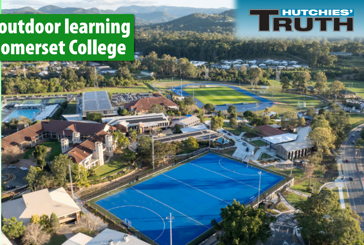
Expansion works at Somerset College on the Gold Coast includes an international-grade hockey pitch with an underground carpark beneath.
